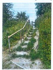
Infrastructure works have begun, and a handrail (*Left.*) has been installed at the entrance from Harbour View Rd- with members of the public already expressing their happiness with it. A stile is next on the list, to prevent any breakages to the fence line in a popular cut-through spot.
